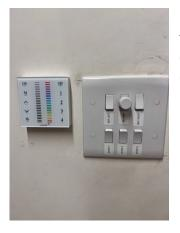
First turn on the light switches on the right-hand panel. This will light the LED strips on the hall struts. On the left-hand panel you can change the colour of these lights by running your finger up and down the rainbow strip.
